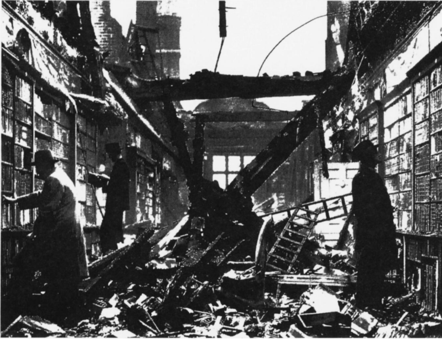
Ruins of the "Holland House" Library in Kensington, London. 1940.
